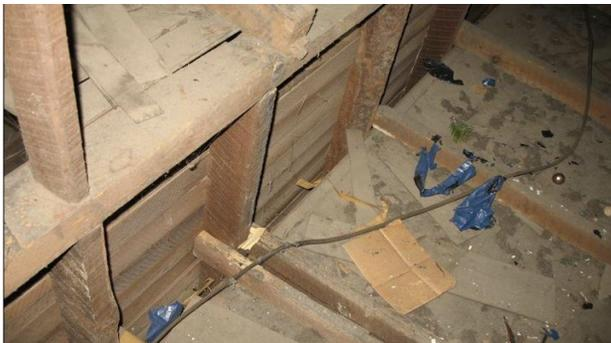
This is an open wall top. Heated air from the living space gets into this wall and then gets into the attic and is wasted. It also delivers moisture to the attic which can cause roof rot and mold. And, it can suck on the combustion appliance zone and cause the appliances to backdraft. Also, cold attic air can drop into the living space through these openings.
