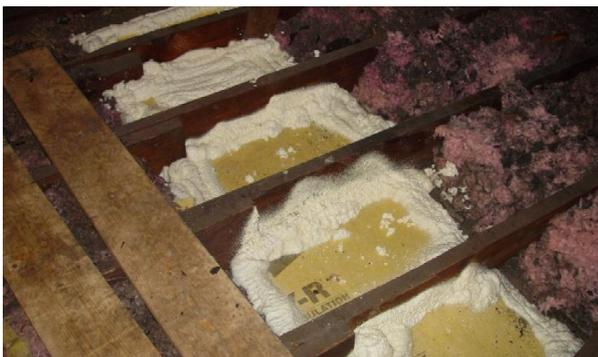
The pressure boundary is re-established by capping this dropped soffit (bulkhead) hole with foam board at the same level as the rest of the attic and air sealing. Insulation will be blown over this whole area, and the old insulation, now.
