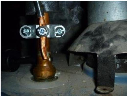
Test smoke isn't going up the chimney, indicating weak draft
